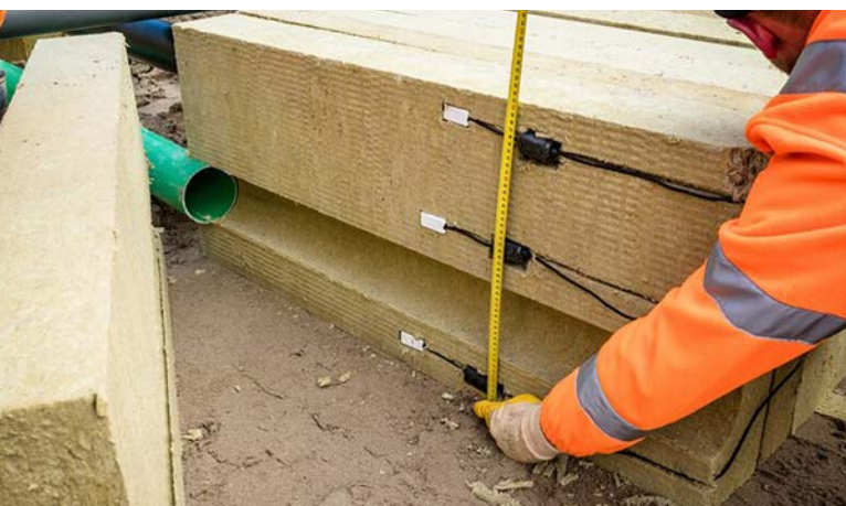
Stone wool in use under a tramline.
