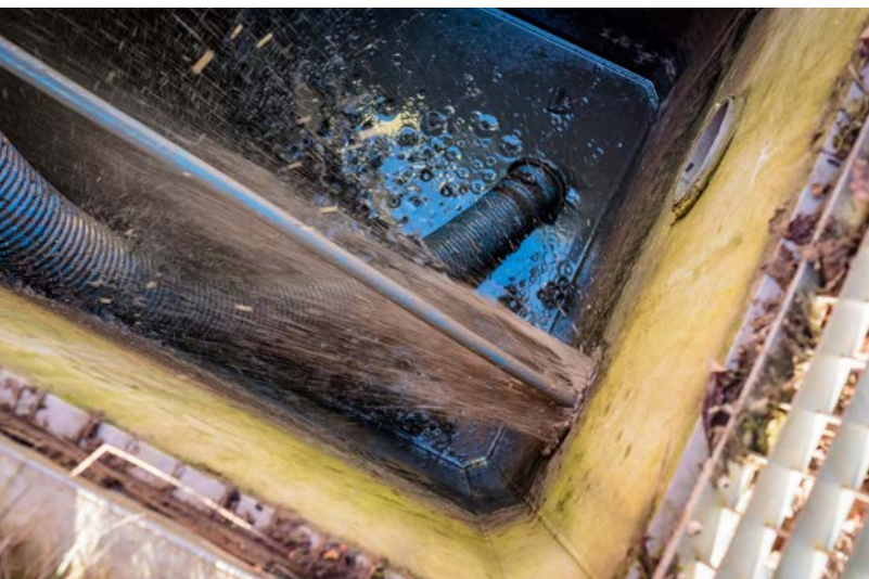
Left: Sediment being removed from the channels. Right: A back-spraying high pressure spray.
