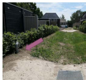
Venting via a gooseneck vent pipe
